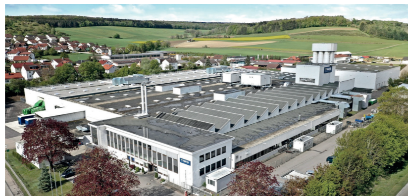
The Varta facility in Dischingen produces around 1.75 billion batteries a year.
